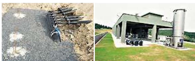
Photo 1,2. Landfill gas production facility, İstanbul
